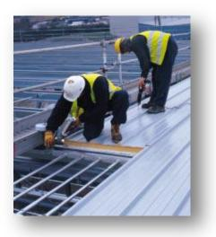
The Rossway Safeway system provides fall protection to the "leading edge"; the open edge that is presented when roof panels are laid in a tier fashion. It also provides protection to the "working edge" the area that is exposed to a fall when the leading edge protection is moved by the tier width of the panel being installed.
